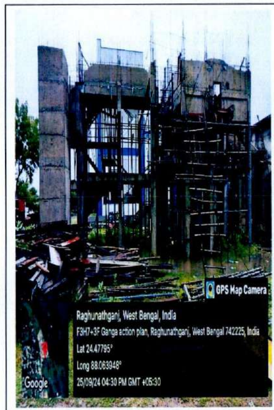
RAGHUNATHGUNJ STP SITE
